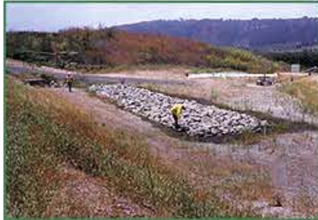
Figure 11. An extended infiltration basin that was constructed by Caltrans, San Diego County Chatsworth Reservoir
