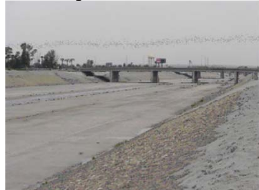
Photo 4.3 Concrete-lined channel along the Los Angeles River
